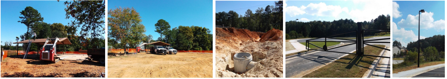
From (L-R) Tearing down the old playground at E.E. Robinson Park in preparation for a new covered pavilion playground. Work at the access road on Hwy 20 for our 90 acres. Finished expanded parking at Gary Pirkle Park.
